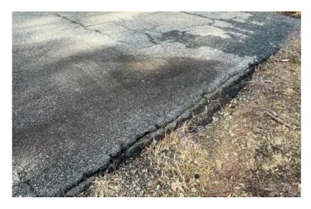
The standard construction of asphalt pavement is compacted soil with four to six inches of well compacted base (i.e., crushed granite) and then asphalt layers totaling three to four inches. The durability of asphalt is determined at least as much by the strength and stability of the soil and base as it is by the quality of the asphalt pavement. The asphalt is in fair condition.
