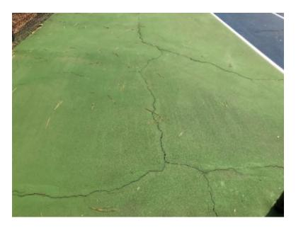
The cracks are easy to repair if a short-term approach is acceptable. Basic crack repair during the application of the colored surface is only effective for about a year before the cracks begin to reappear. There are crack repair techniques that are guaranteed for five years, but the cost is high (between \$11 and \$15 per linear foot). The cost of this type of crack repair can be prohibitive if there are numerous cracks.
