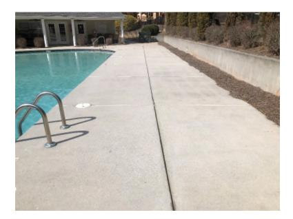
Some Associations will have a surface coating applied, but that is often not cost efficient because the coating is expensive (about 40% of the cost of a new pool deck), entails some additional maintenance expenses, and can flake off if it does not bond properly. Also, as problems develop in the original deck (such as cracking), that causes issues in the coating.
