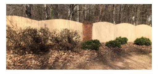
The fencing appears to be original with the property which would make it about twenty-five years old. Some of the pickets are warped and others are deterioration on the top edge as seen in the next photo.
