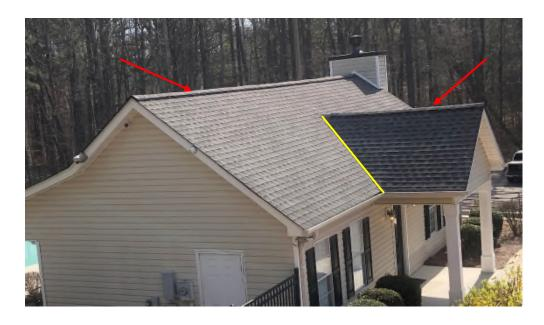
The roof of the clubhouse has shingle over ridge vents (indicated in the previous photo by the red arrows), which are the most effective in allowing warm air to escape the attic. A properly installed ridge vent with proper air intake provided by your perforated vinyl soffit increases energy efficiency and prolongs the life of the roof.
