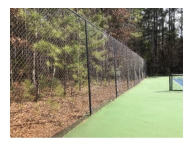
The poles should last indefinitely, but the fence fabric will need to be replaced. The existing fence is good quality, but at the tennis courts, there is only has a tension wire to hold the chain-link fabric at the bottom. This can be unsatisfactory where there is vigorous play (i.e., with people crashing into the fence). A horizontal pole at the bottom can sometimes help keep the fence from curling.
