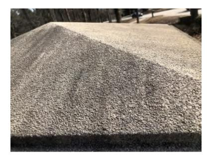
The largest single item in this category is the replacement of the pool deck at a cost of about \$40,000. Pool decks generally have a life of thirty to forty years depending on the quality of the original concrete and the workmanship. Replacing the pool deck is usually done when the pool is being re-plastered because the demolition of the pool deck sends a lot of debris into the pool. The pool deck is in good condition and it is unlikely that it will be replaced in this twenty-year period.
