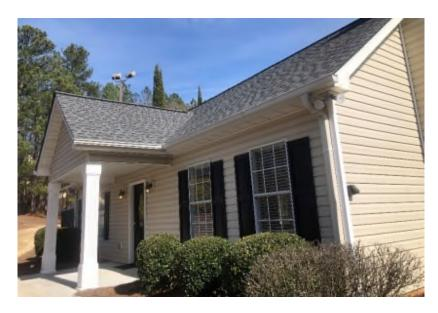
The surfaces that require painting are the exterior doors, the door jambs, the wood front columns, vinyl shutters, the aluminum rear columns (including the wood posts at the pool fence), and the chimney pan and flue. The paint on the door jambs at the storage room is failing (seen in the photo on the left), and the door jamb is deteriorating at the bottom. The paint on the precast aluminum base for the rear column seen in right photo is failing.
